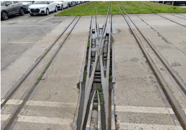
Work to repair rail siding n° 13
