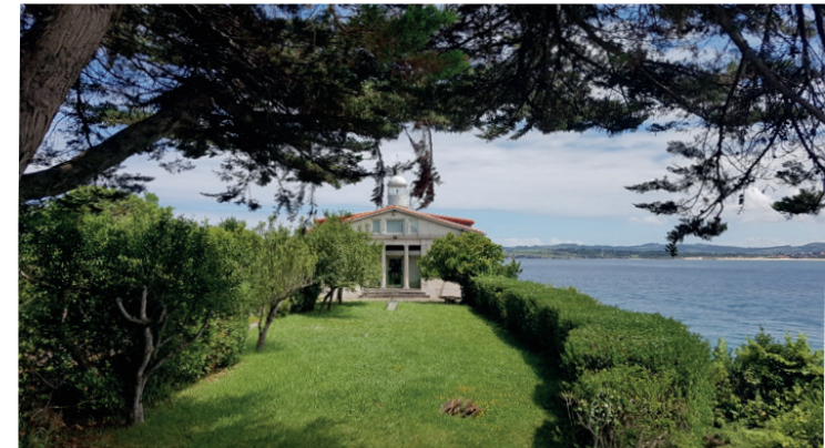
Installations of La Cerda Lighthouse. Headquarters of the Santander Port Lab.
